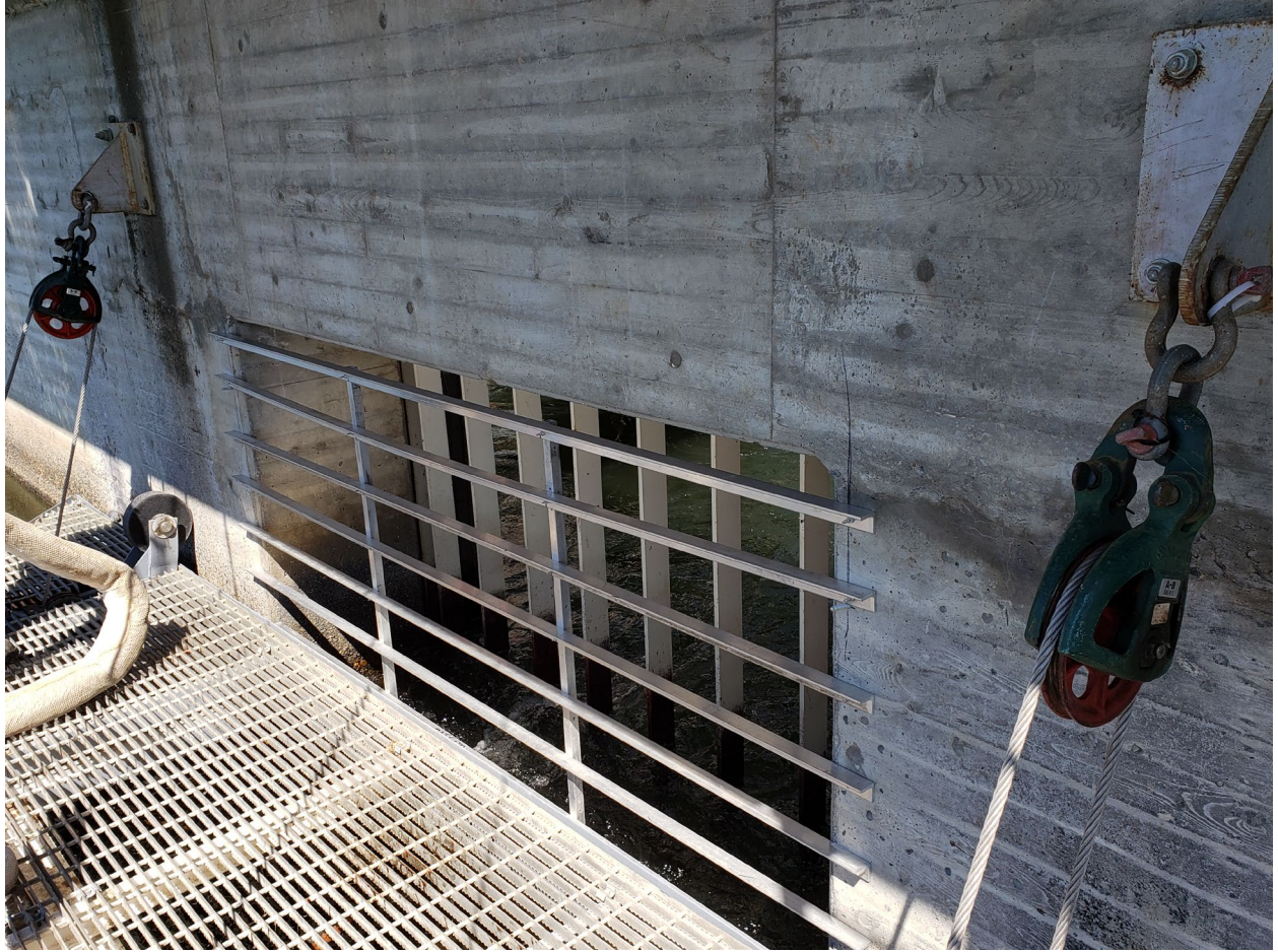
View of exclusion from outside.
