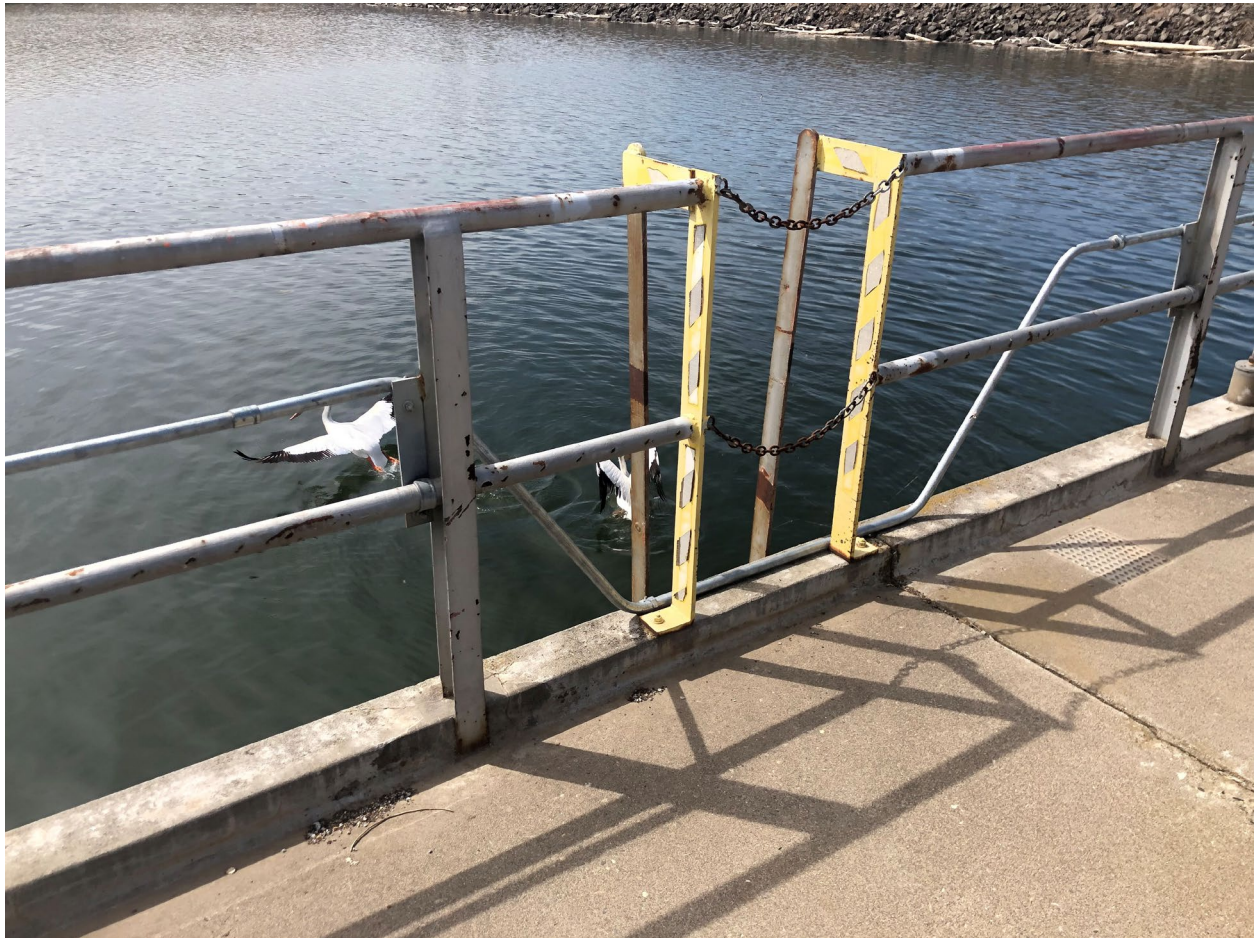
Pelicans outside ladder near floating trash rack.
